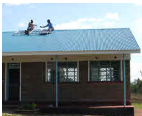
Electricians installing solar power
